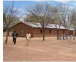
Roof St. Andrew's Church
